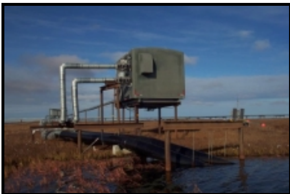
Figure 2. Pumphouse at lake L9312.
