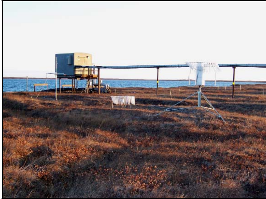
Figure 2. Newly relocated meteorological station at L9312. Photo by D. Reichardt.
