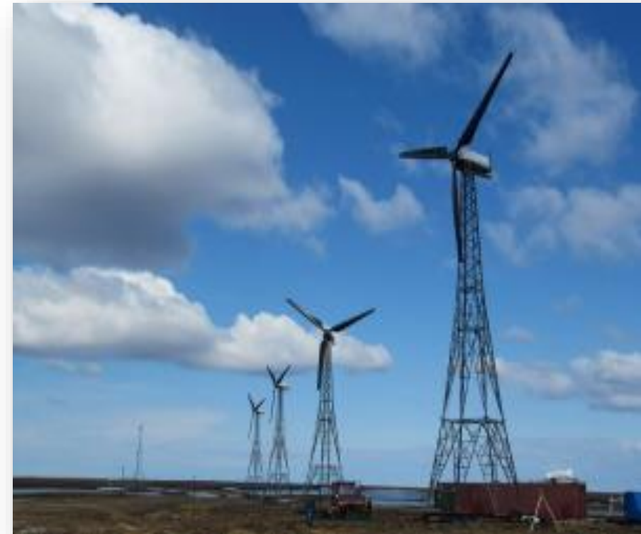
5 - 95 kW Windmatic direct drive wind turbines (30-40% wind penetration annually)
