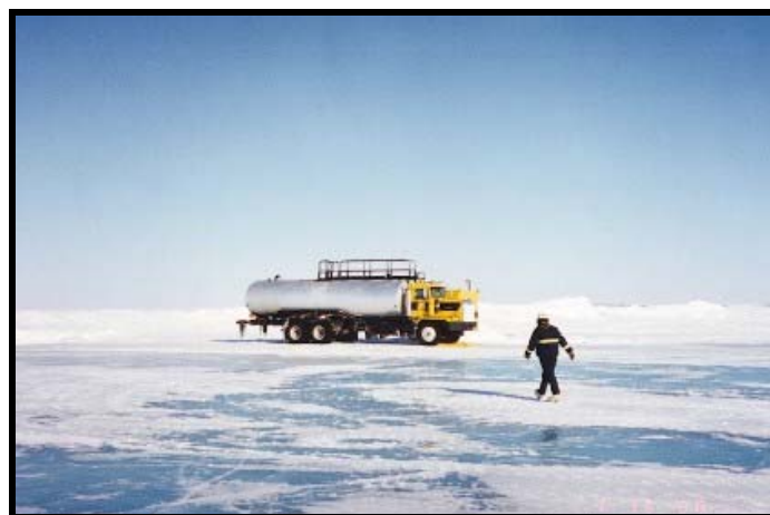
Figure 4: Ice road construction begins when the active layer (seasonally frozen ground) is satisfactorily frozen. Snow is packed and then pumped water is sprayed onto the snow surface until a sufficient road thickness is attained (photo — W. Morris).
