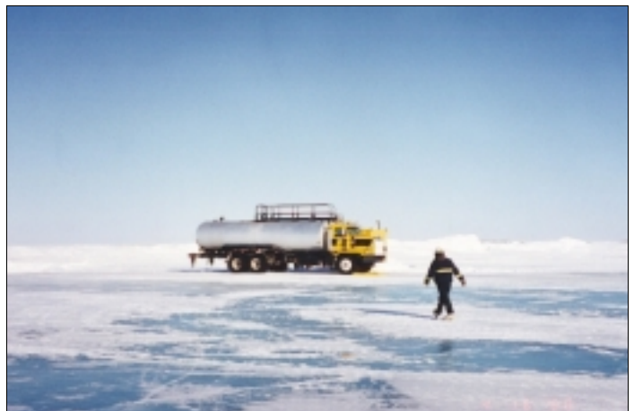
Figure 4: Ice road construction begins when the active layer is satisfactorily frozen. Snow is packed and then pumped water is sprayed onto the snow surface until a sufficient road thickness is attained (photo — W. Morris).
