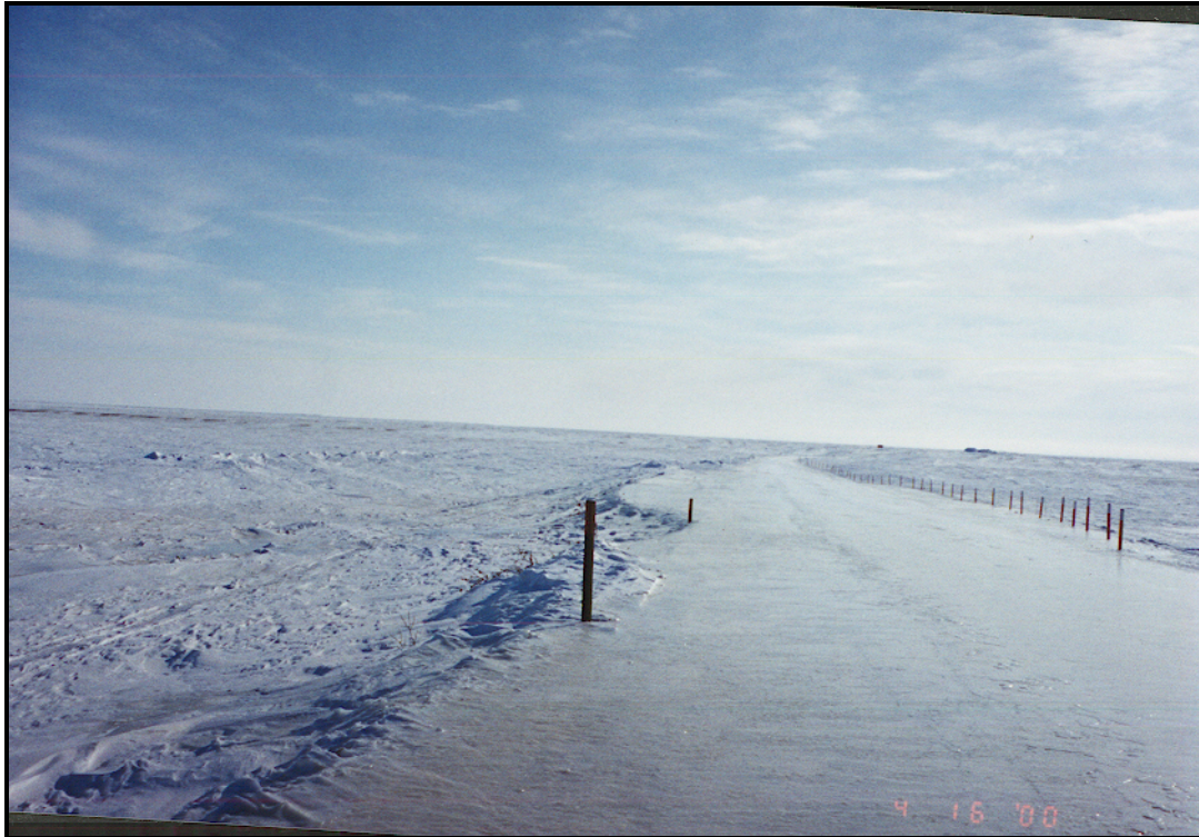
Figure 3. A completed ice road looking northeast toward the Alpine Oil Field (photo by Bill Morris, Alaska Department of Natural Resources).
