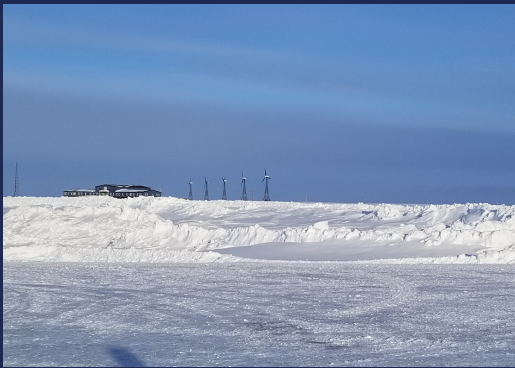
In Kongiganak, five 95 kW wind turbines spin year-round, producing electricity to power the community. Excess energy is used to heat thermal bricks, reducing households heating costs.
