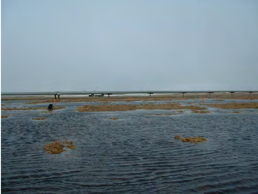
Figure 76: Photo of outlets 1 and 2 at Lake K113C.
