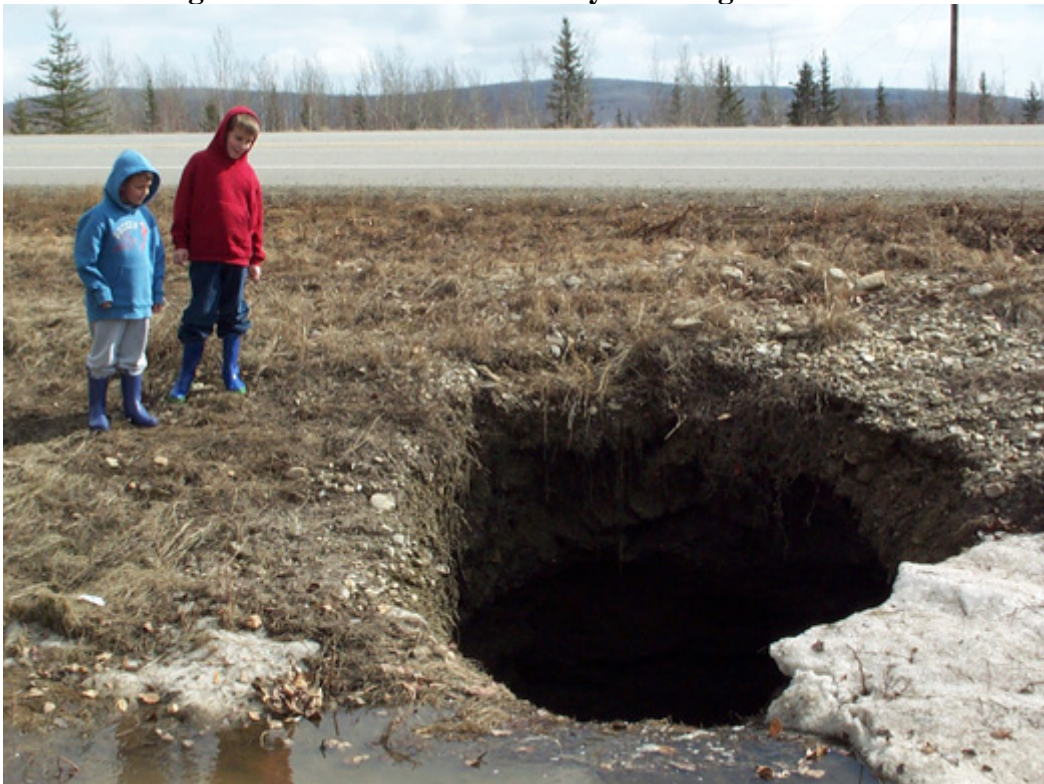
Figure II-3. Sinkhole Created by Thawing Permafrost
